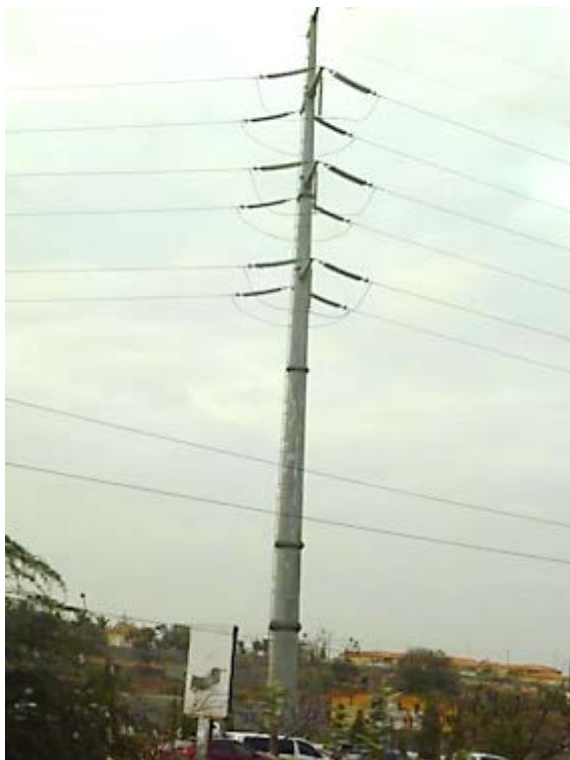
Figure 7-9 220 kV steel pipe tower (tension)
