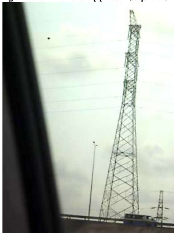
Figure 7-12 220 kV steel angle tower
