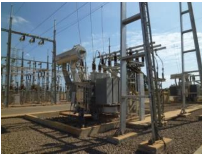
Figure 7-14 66 kV/15 kV transformer made in China
