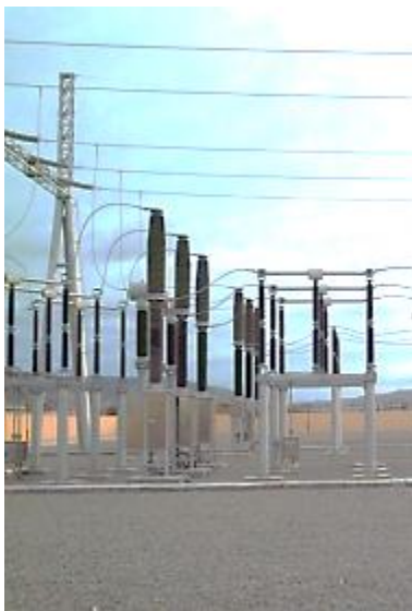
Figure 7-16 220 kV vertical type gas-insulated circuit breaker
