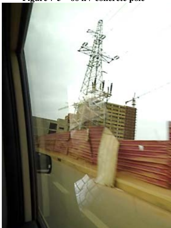
Figure 7-7 60 kV underground cable branch tower
