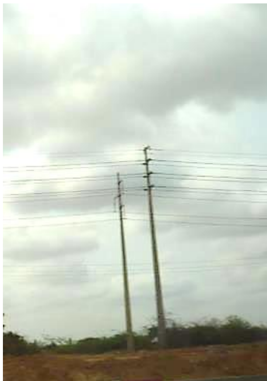
Figure 7-5 66 kV concrete pole
