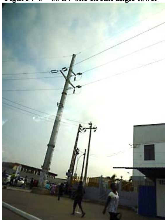
Figure 7-8 60 kV steel pipe tower
